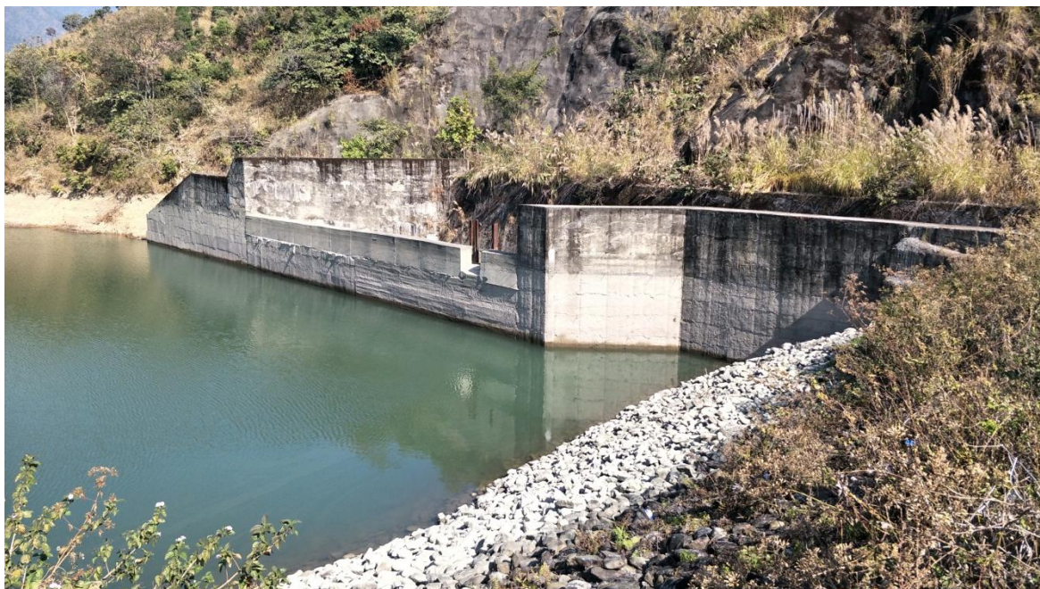
Photo 2: Spillway of Singda dam
