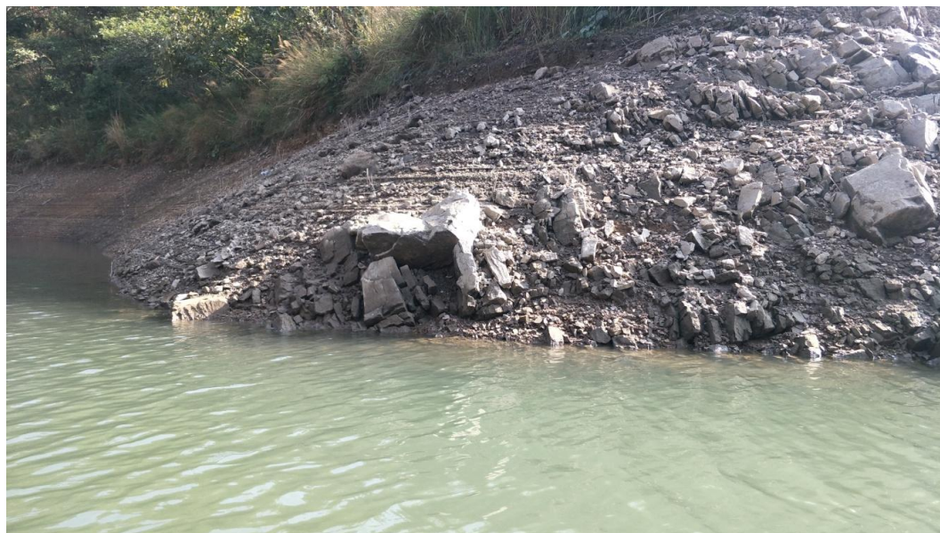
Fig. 18: Soil erosion at river left bank hill.
